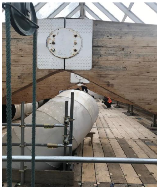
Access: Removal of ducting and apex connections
