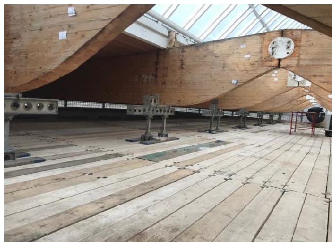
Structure: Access to timber beams and connections
